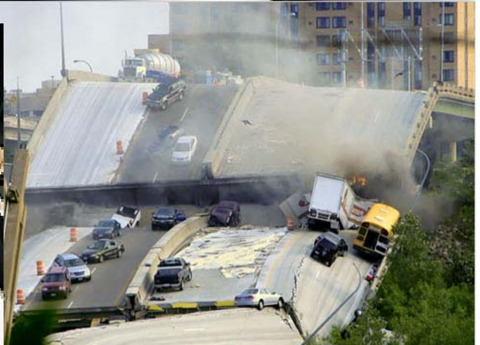
A Broke & Broken System
